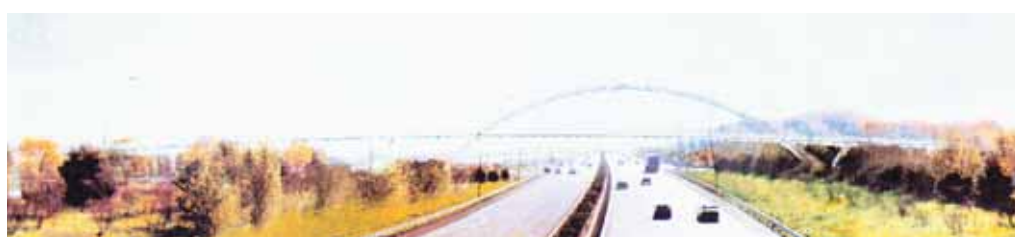
Figure 7 Viaduc Rocade Ring road viaduct
